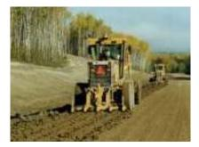
The road is scarified to break the soil into lumps small enough to be further broken down by harrows.
