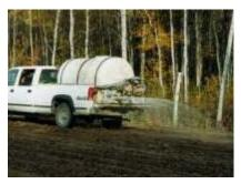
Following the scarification RoadPacker Plus is then applied to the soil. The most efficient method of doing this is by spraying a diluted mixture directly onto the soil.
