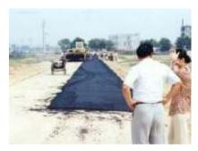
The surface can now be left as is, giving a durable, low maintenance, cost efficient running surface or it may be covered with an asphalt covering. Either a hot asphalt or a cold mix may be applied, according to the specification and application of the job.
