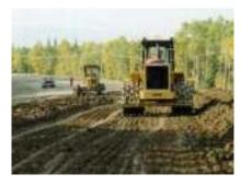
Upon completion of the mixing, compaction begins. The initial compaction is usually carried out with a pads-foot vibratory compactor.
