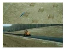
This gives very thorough compaction, leaving the surface very hard and completely waterproof. The surface can now be smoothed using rubber wheeled rollers.
