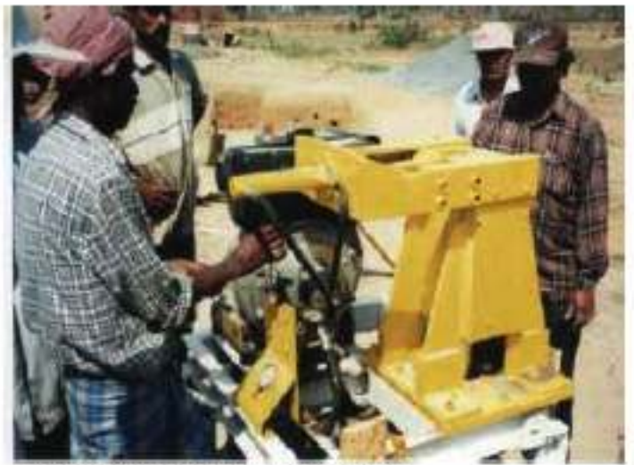
Pressing the compaction lever
