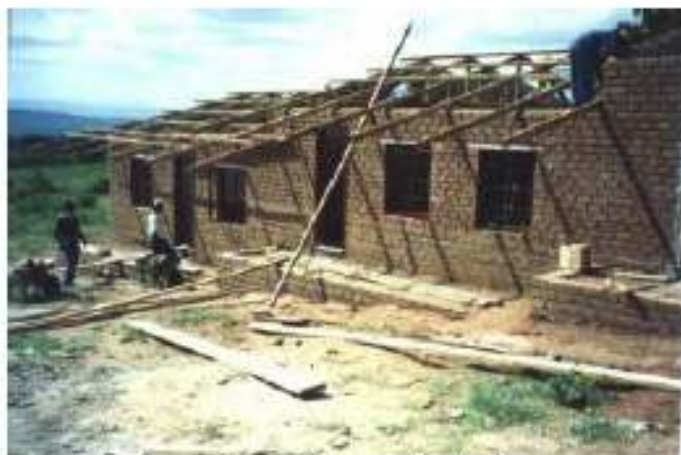
The Roof may be easily applied using conventional methods or by using our Agritile technology utilising the insitu soil, as with our soil blocks.
