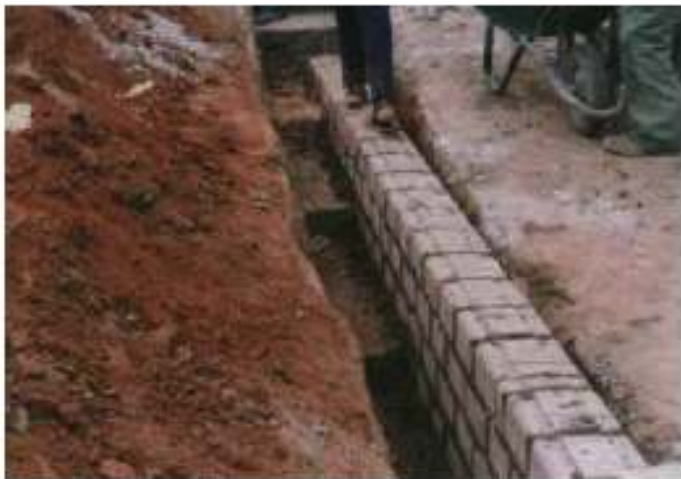
Foundations are made using the same blocks reinforced with mortar, building then commences above by dry stacking the blocks one on top of the other.
