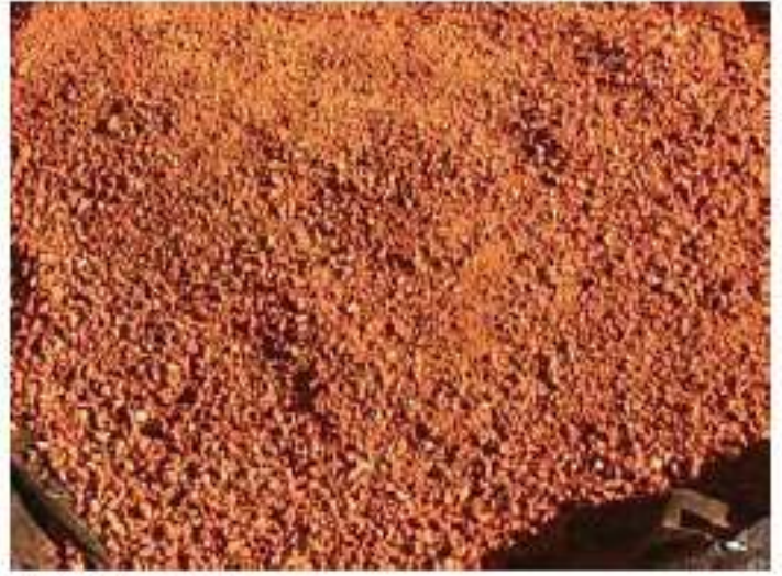
Soil being crushed before mixing with chemical
