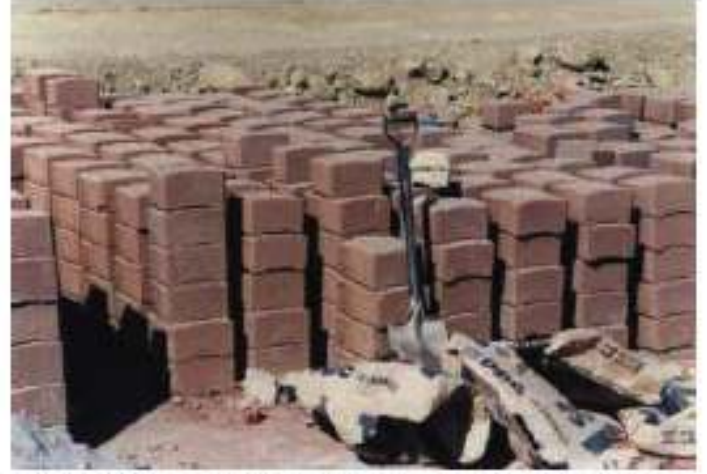
Blocks are then stacked for curing for a short period of time and then building may commence
