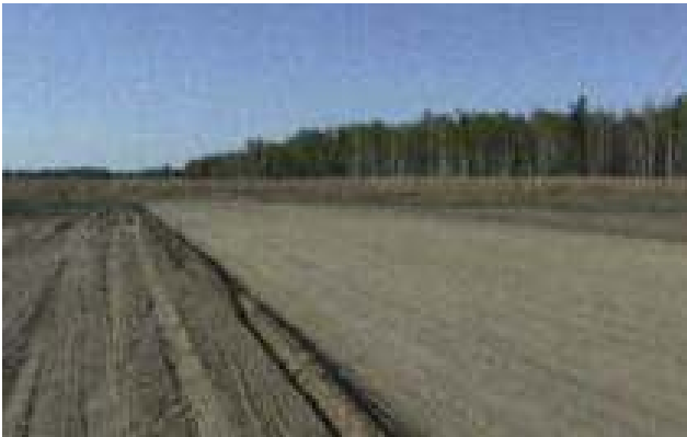
This is the same airstrip after it has been treated and packed with RoadPacker Plus
